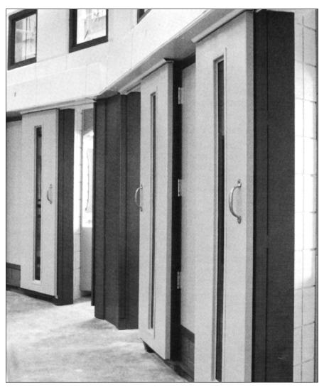
In event of power failure, all doors remain in a fixed position, and must be operated mechanically. Doors are freewheeling when released.
