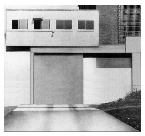
**Bi-parting Door Model:** Secured by cremone bolts operated by prison paracentric key. (See Mechanical Lock Section for details.)
